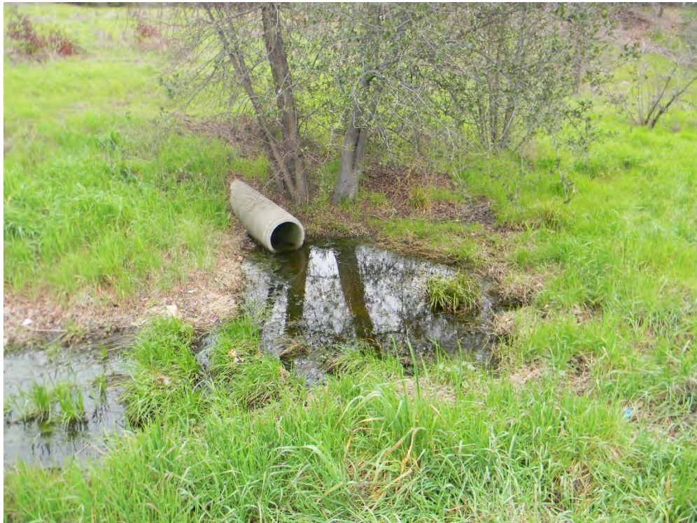
6. Southeastern part of site, view to northeast showing culvert outfall along smaller of two intermittent streams.
